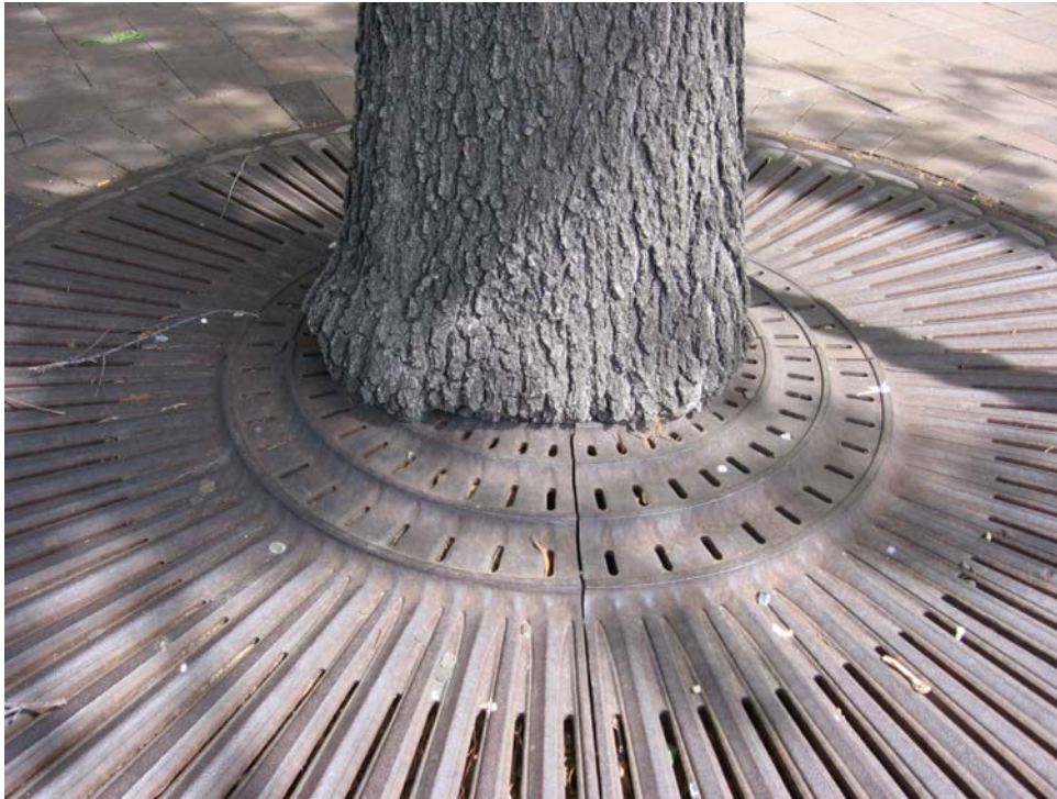
Tree growing into tree grate, restricting growth and will almost certainly lead to mortality of the tree (photo taken from The Case For Big Tree Openings | DeepRoot Blog )
